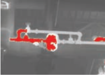
Figure 5-60. A properly working steam trap should be warmer on the steam side and cooler on the condensate side as is the case in this image.
