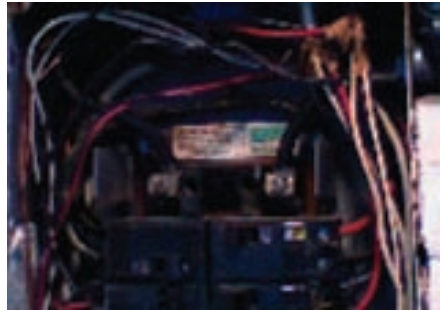
Figure 5-7. A high-resistance connection or component malfunction within a residential circuit breaker is easily seen in the thermal image, but not in the visible light image.
