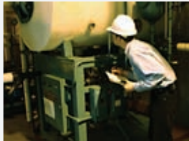
Figure 10-1. Maintenance technicians routinely check the appearance and sounds of operating equipment by conducting visual and auditory inspections.
