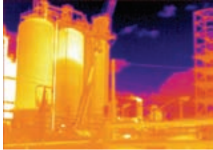
Figure 5-61. Liquid levels in storage tanks are easily seen with a thermal imager when conditions are optimal.
